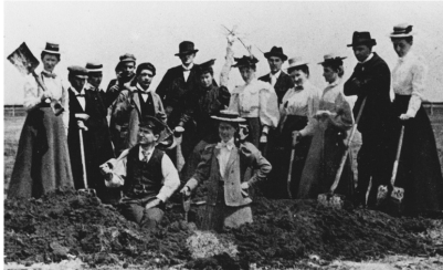
Ground Breaking Ceremony
