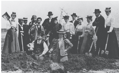
Ground Breaking Ceremony
